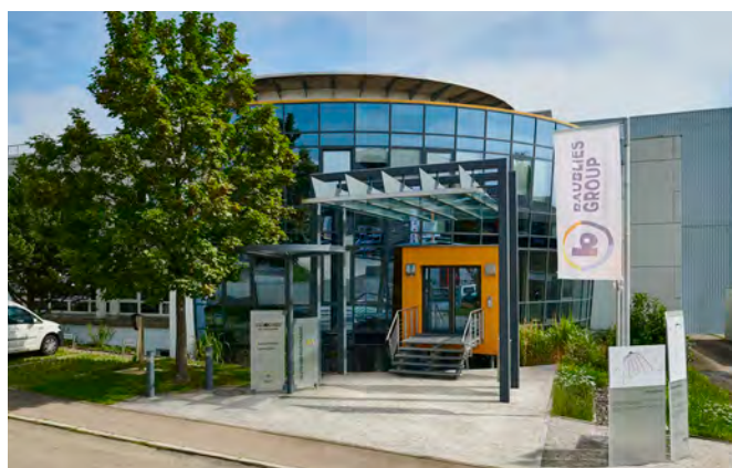
Wagner Tooling Systems Headquarter in Pliezhausen
