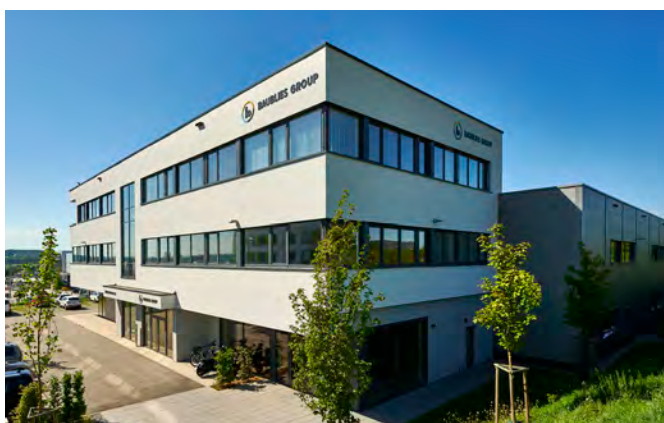
Baublies Headquarter in Renningen
